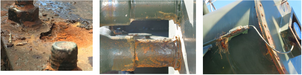
Figure A-3: 2017 Inspections on various components
