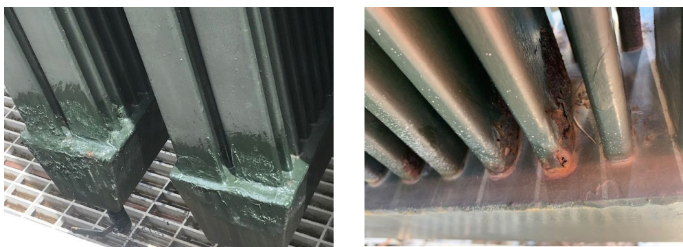
Figure B-3: 2021 radiator repair and 2023 Inspection on radiators
