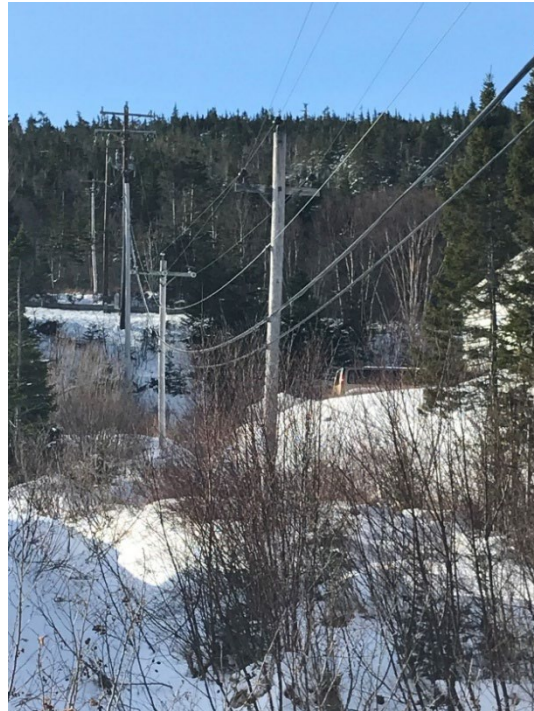
Figure 5 - Offroad section of Feeder Trunk
