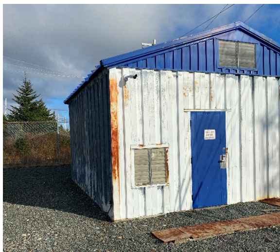
Figure A-7: BLK Control Building
