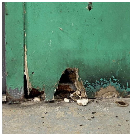
Figure A-8: BLK Control Building
