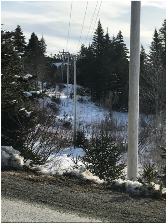
Figure 4 - Offroad section of Feeder Trunk
